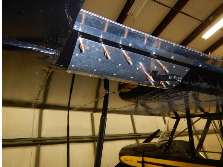
Figure 6: Rivet doublers to false spar
